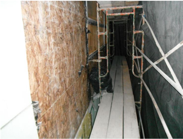
Stucco Demo'd and some sheathing removed
